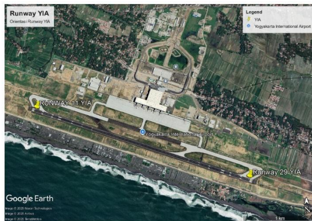
Gambar 1. Landasan pacu ( Runway ) Bandara YIA
